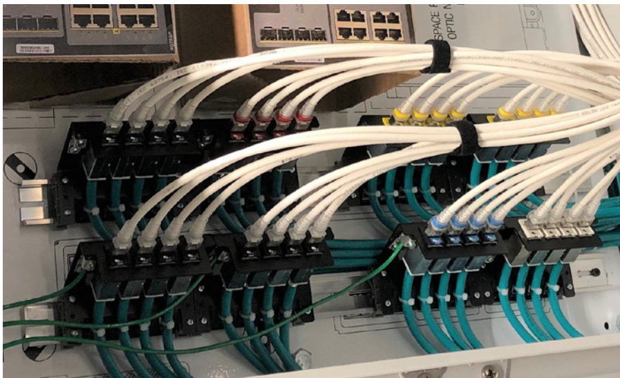
DIN Rail installations using shielded cabling supports PoE applications.
